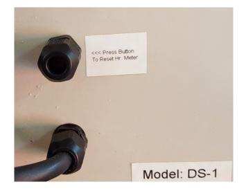
Your DS system is fitted with a digital hour meter to monitor run time. If the system is turned off or power fails the e-prom memory will remember the last reading and restart at the last reading. After 9,000 hours replace the UV Lamp and then use a pen tip to press the button seen in the photo above. Confirm the reading resets back to zero.
